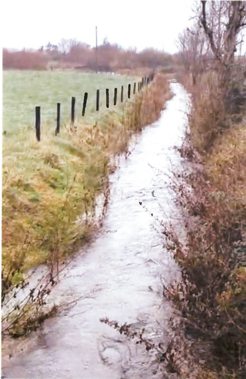
Figure E3. 2024 high flow in the existing drainage channel directly across the road from the observer's property, beside the proposed Location 17 sweep/overrun area.
