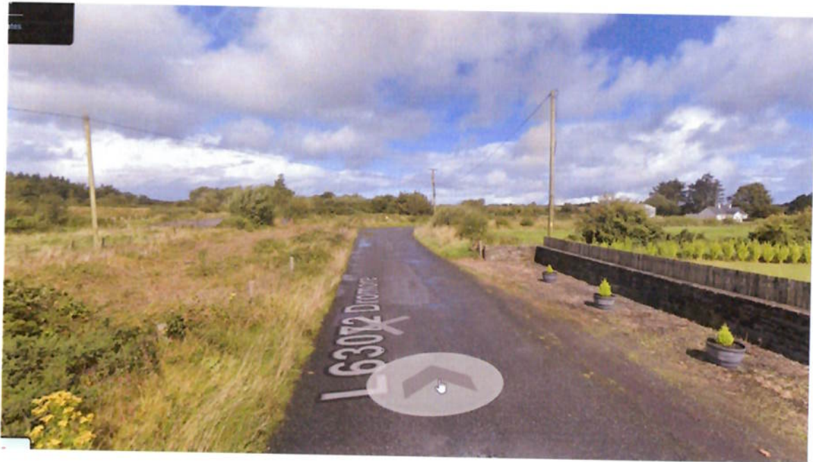
Figure G1. Street View imagery showing the sequence of existing roadside utility poles and overhead services along the approach to Location 17. The imagery is used to establish the presence and general roadside position of the utility infrastructure.
