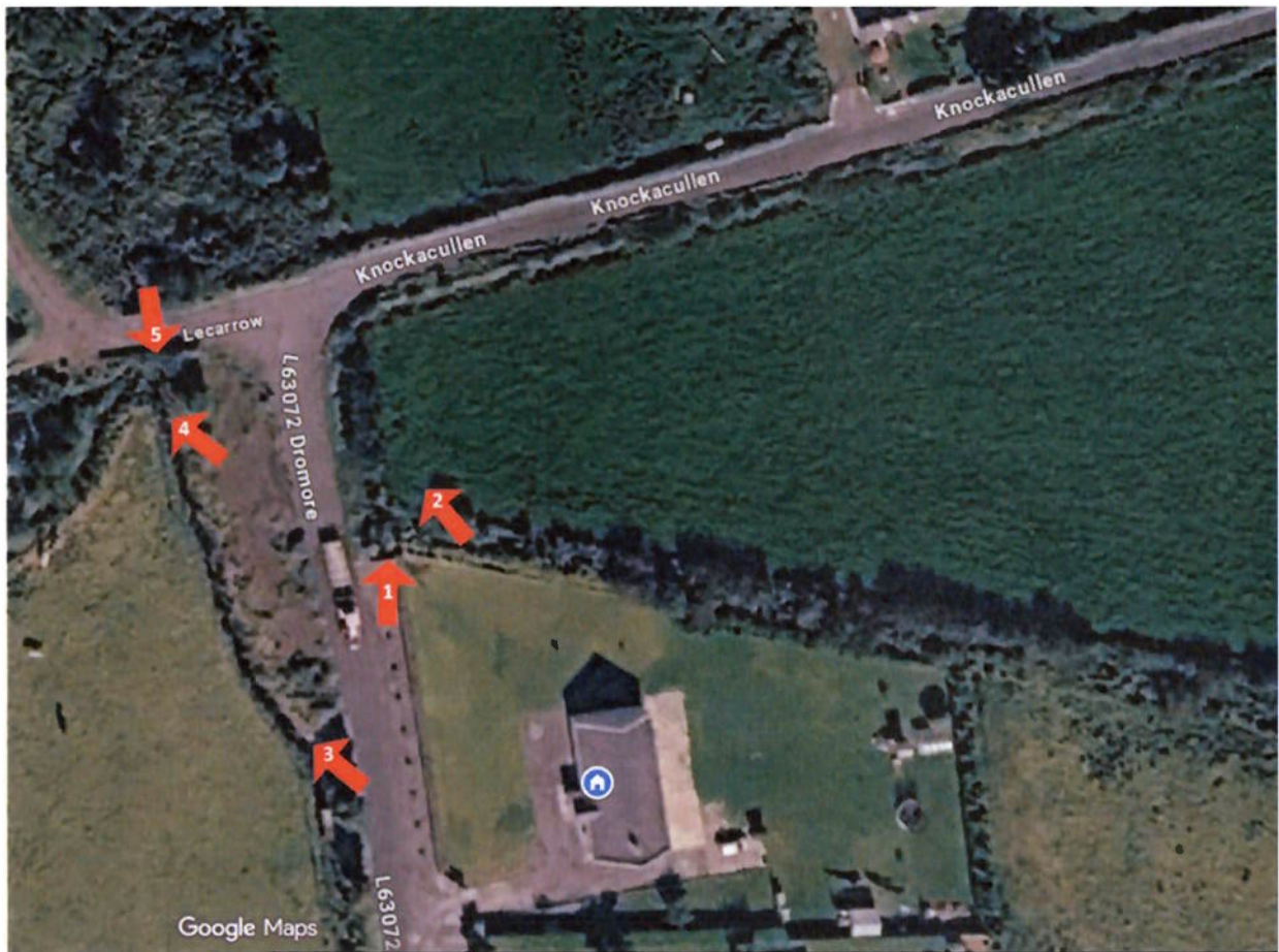
Figure E6. Approximate locations of the 2024 flooding/high-water photographs shown in Figures E1–E5.
